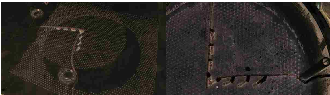
Figure 3.9: Geogrid installation
